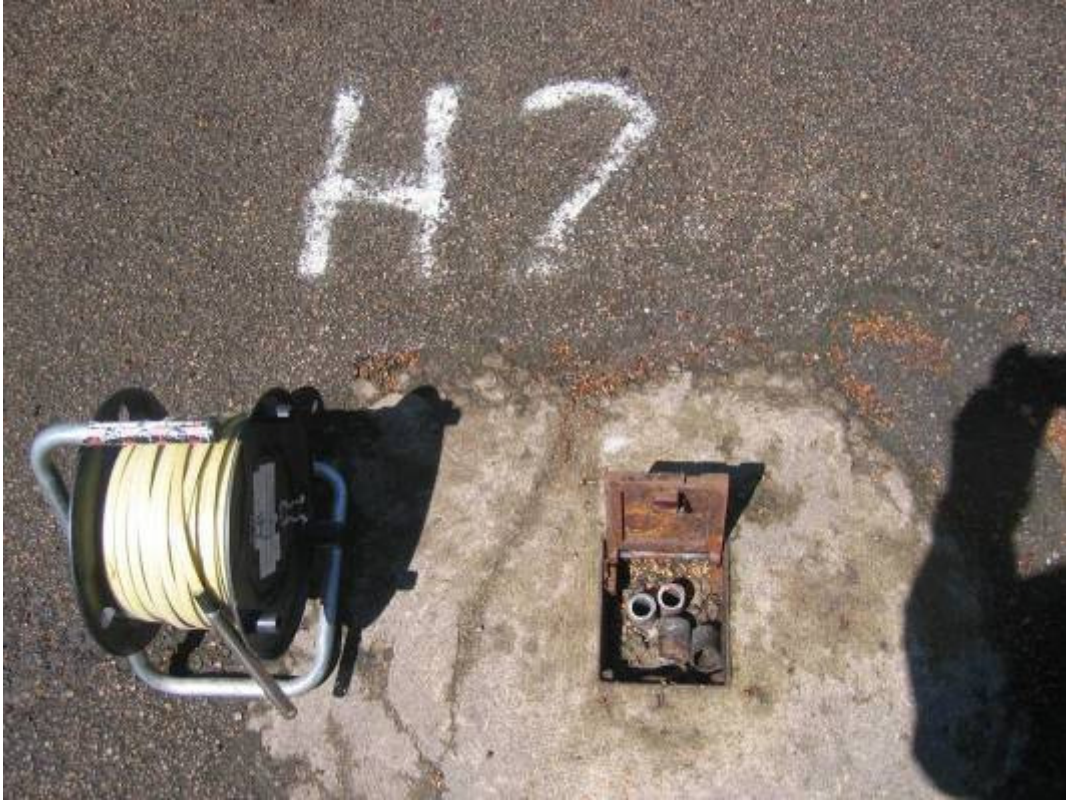
Plate 31 Scarborough South Cliff H2
