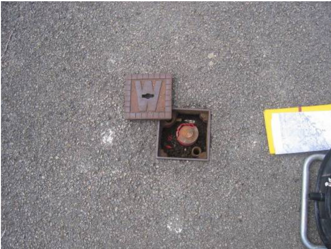
Plate 28 Scarborough South Cliff Bh2
